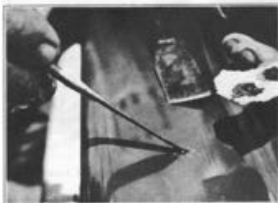
Figure 2J-3. Filling Hole or Scratch
