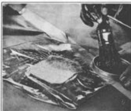
Figure 2J-10. Applying Resin to Mat
