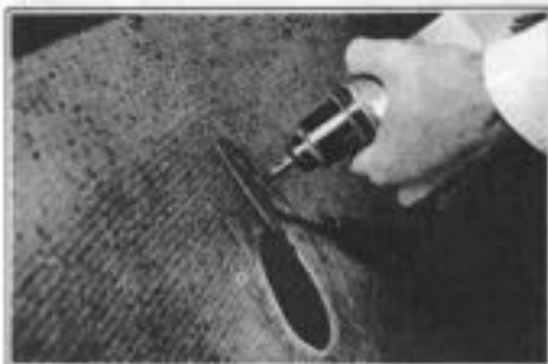
Figure 2J-8. Rough Sanding Inside Surface
