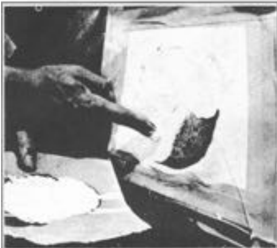
Figure 2J-14. Working Gel Coat into Patch
