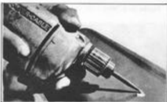
Figure 2J-1. Roughing Damaged Area
