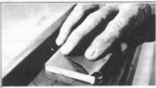
Figure 2J-6. Sanding Patch
