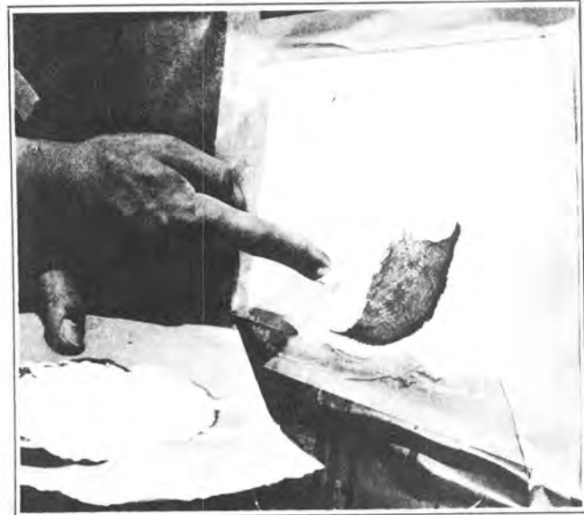
Figure 4-14. Working Gel Coat into Patch
